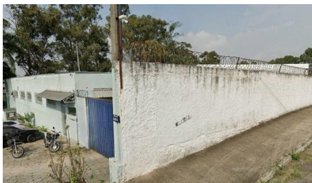
Rua Major Vieira
